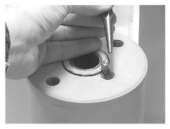
**19.** Insert the set screws (113) over the lock pins. Tighten them to 25 in. lbs. (2.825 Nm).
