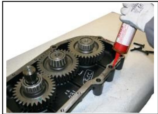
3:16 Apply sealant to the mating faces of the front and rear casing.
